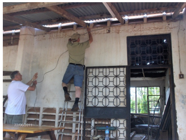
Dave and Tom installing outlets
