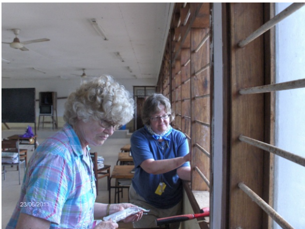
Deloris and Christine repair window hinges.
